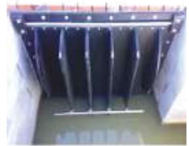
Clapet in polietilene "HDPE-S" flap valve
