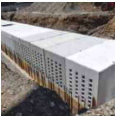
Scatolari e sistemi di drenaggio in cemento Preformed units with rectangular section and stormwater infiltration system
