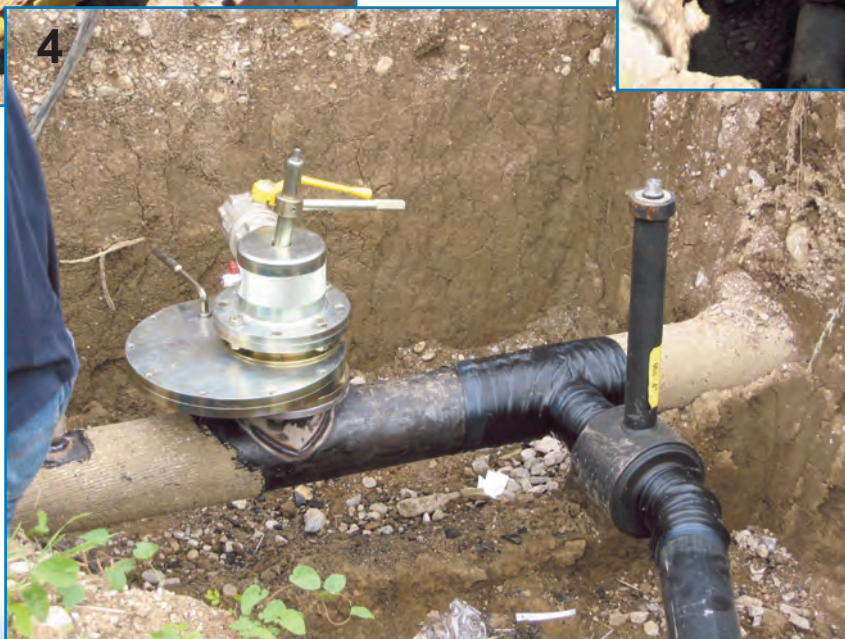
Foto 4 Tamponatrice DN 6" Plugging machine DN 6"
