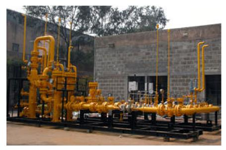
We provides Skid-Mounted Systems, each engineered to our customer's exact requirements for Natural Gas Metering, Pressure Regulation, Conditioning and Control. These skids have been supplied to, Gas Distribution / Gas Transportation Companies and End Users.
