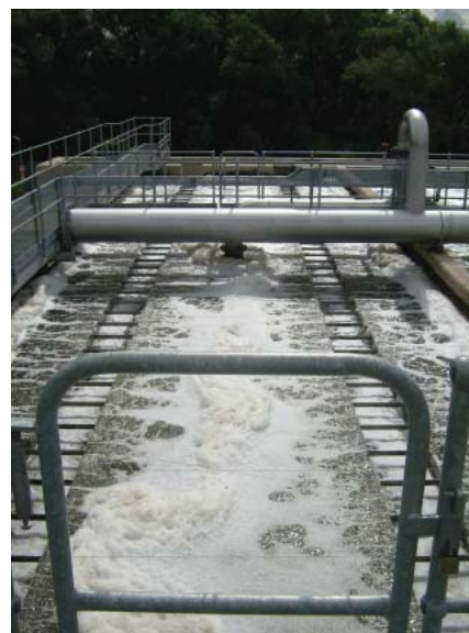
TETRA® NSAF (Nitrifying Submerged Aerated Filter)
