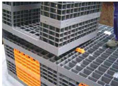
Accoppiamento celle in verticale sulla clip Coupling the cells vertically at the column/clip
